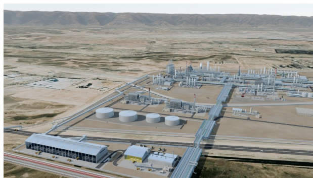
Figure 11. Delayed coker, the two hydrogen plants and sulphur recovery
