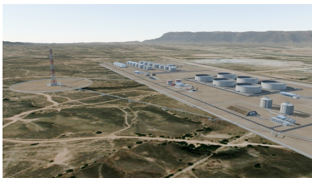
Figure 12. Refrigerated and mounded LPG storage and the 150 m elevated flare
