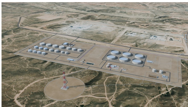
Figure 10. Tank farm on the storage lease: six 116,000 m 3 crude tanks, product and LPG storage
