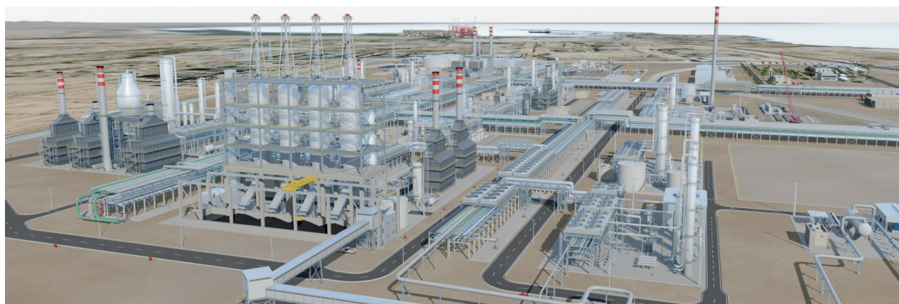
Figure 18. The delayed coker and main pipe racks from the west, with the Port of Salah on the horizon (concept render)
