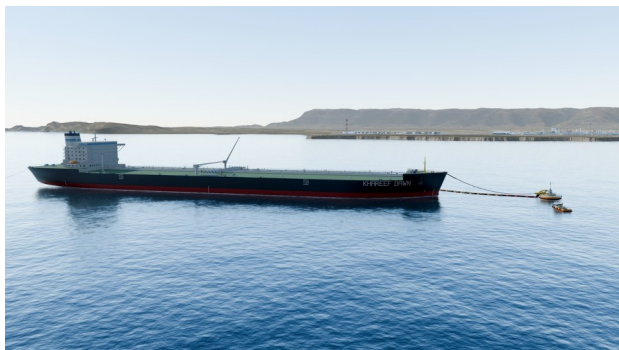
Figure 7. Crude import: a VLCC moored at the single point mooring
